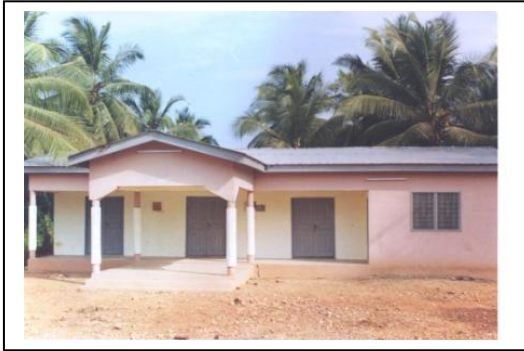
Facilities for the water project and Word Alive Offices
