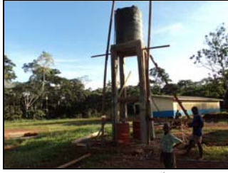
New water tank
