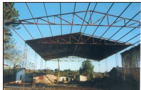
Sports Center under Construction, Argentina
